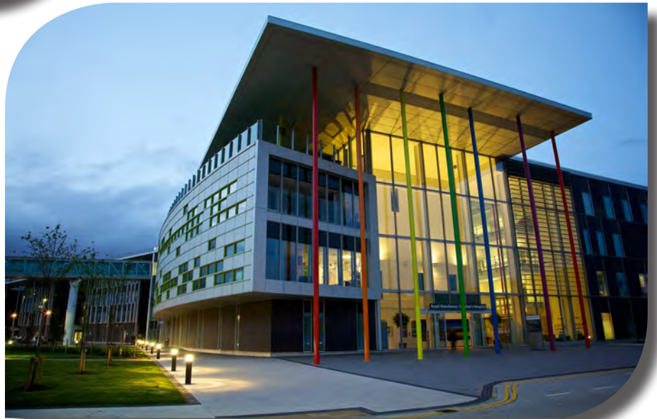
Royal Manchester Children's Hospital (Architect: Stantec). ©Gregory Harding
